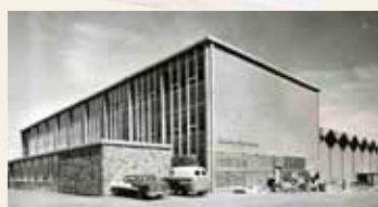
Schafer Hall completed in 1961
